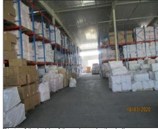
Photo of the inside of the main production hall Finished product warehouse.JPG
